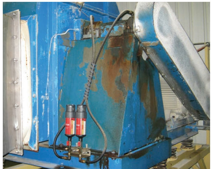
Industry: Power Plant Application: Fan / blower bearings Lubrication system: perma STAR VARIO Installation solution: Remote mount
