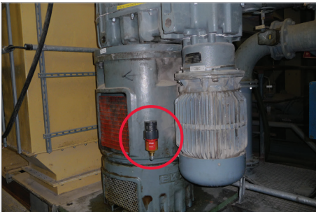
Industry: Power generation
